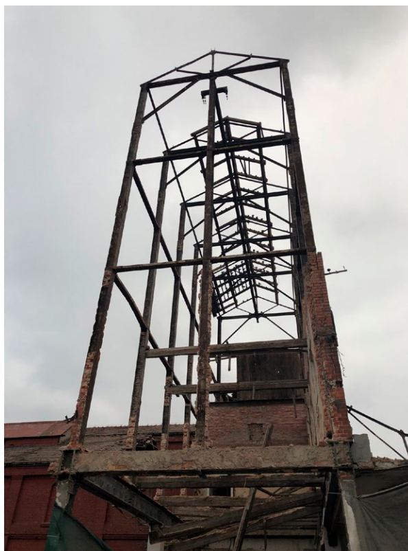
Fig. 5. The high section during the demolition of the deformed and cracked walls with visible corroded steel structure; photo by P. Paradziński.
