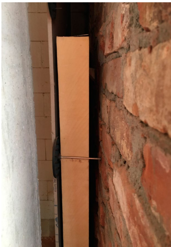
Fig. 9. Thermal wall insulation installed from the inside; photo by P. Marciniak.
